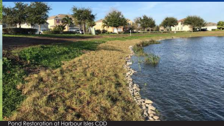
Pond Restoration at Harbour Isles CDD
