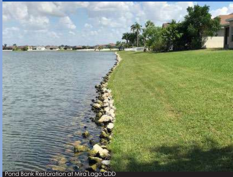
Pond Bank Restoration at Mira Lago CDD
