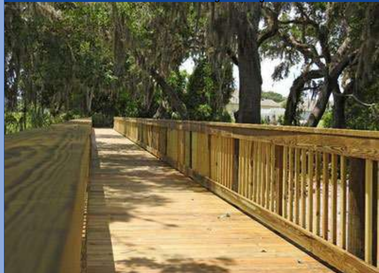
Pedestrian Boardwalk at Oak Creek CDD
