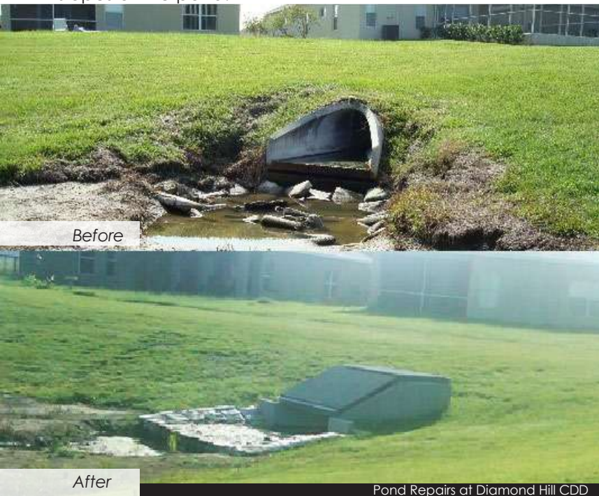
Pond Repairs at Diamond Hill CDD
